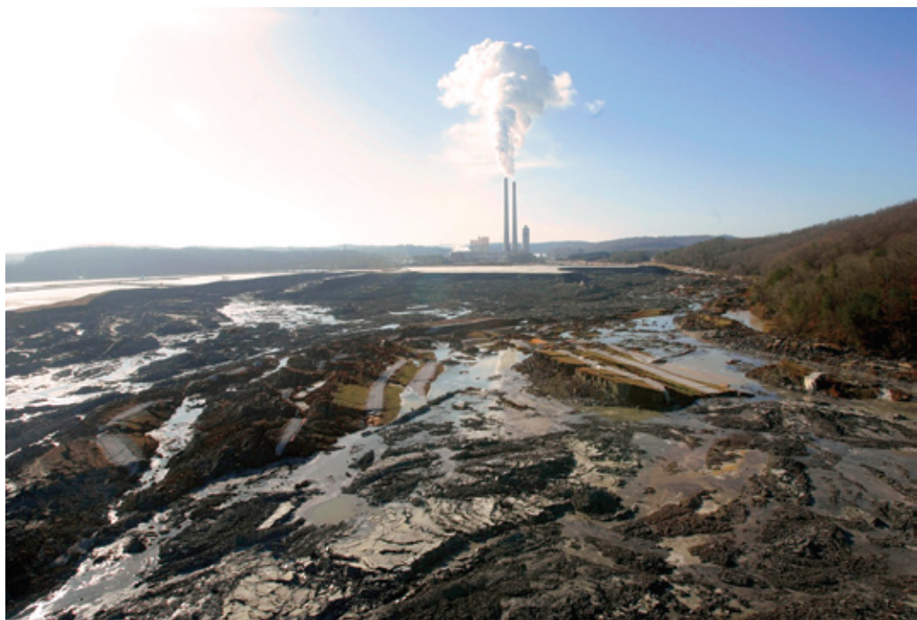
An aerial view shows the aftermath of a retention pond wall collapse at the Tennessee Valley Authority's Kingston Fossil Plant in Harriman, Tenn. (AP Photo/Wade Payne, File)
